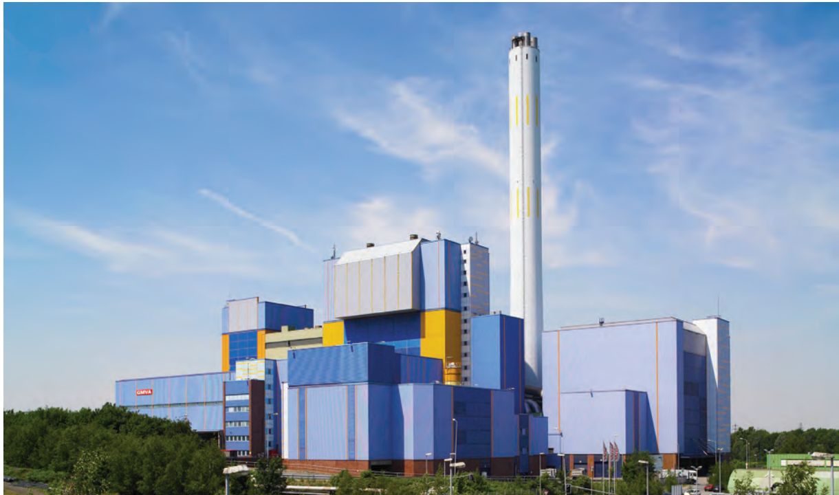
Germany has been using waste to generate electricity since the early 1990s. Pictured is REMONDIS' Oberhausen plant.
